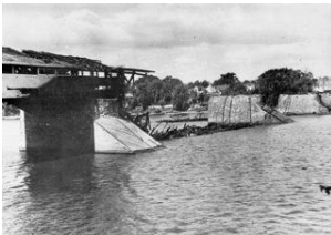
Bridge after Fire
