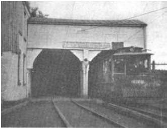
Trolley exiting Bridge
