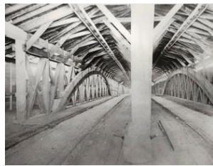
Inside original Bridge
