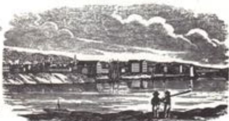
Northwestern view of Lansingburgh
