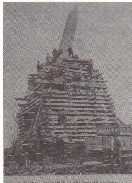
THE WOOL MONUMENT, IN PROCESS OF ERECTION.
